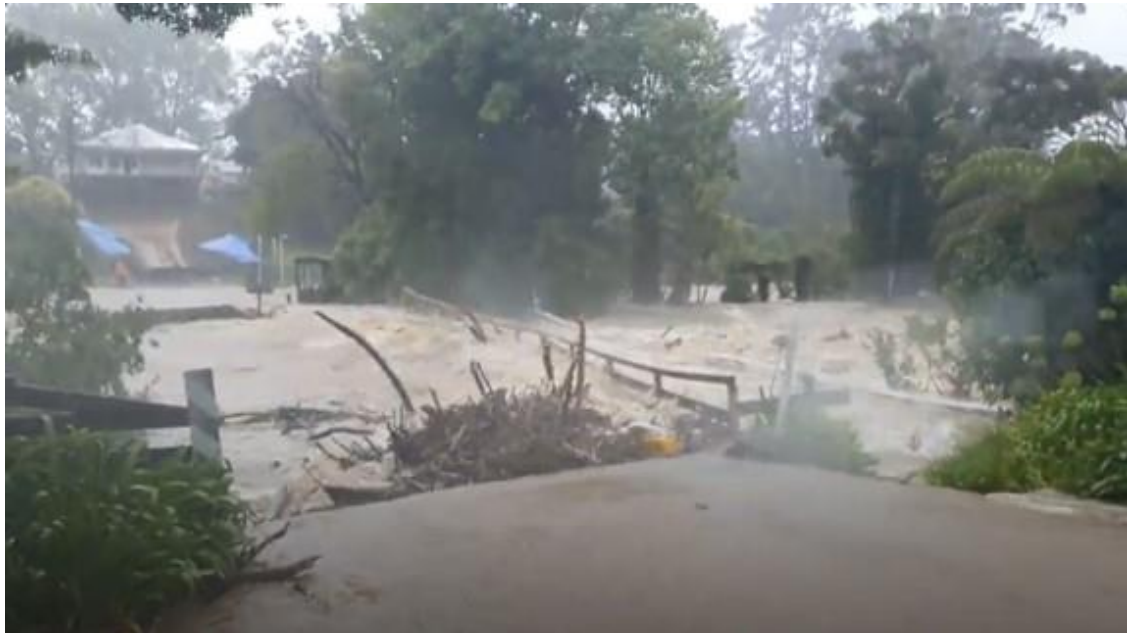
Mill Flat Road Bridge
