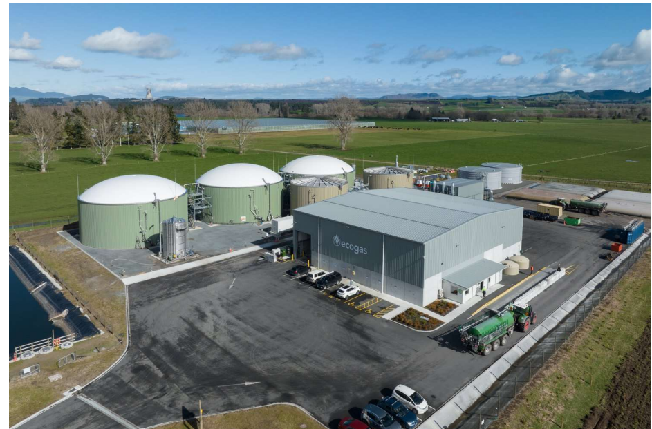
Biogas plant in Auckland
