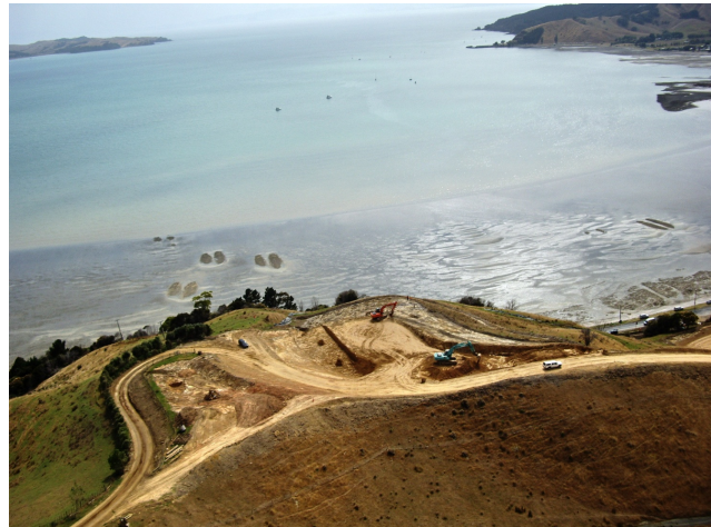
Figure 10: Earthworks Commencement January 2009
