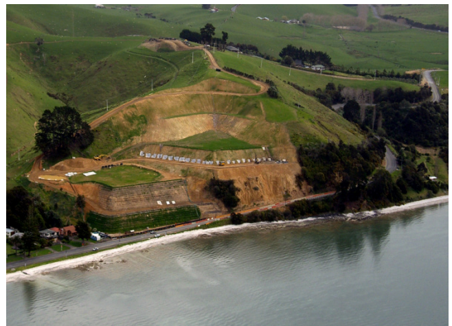
Figure 14: Rock Anchors Being Installed August 2009
