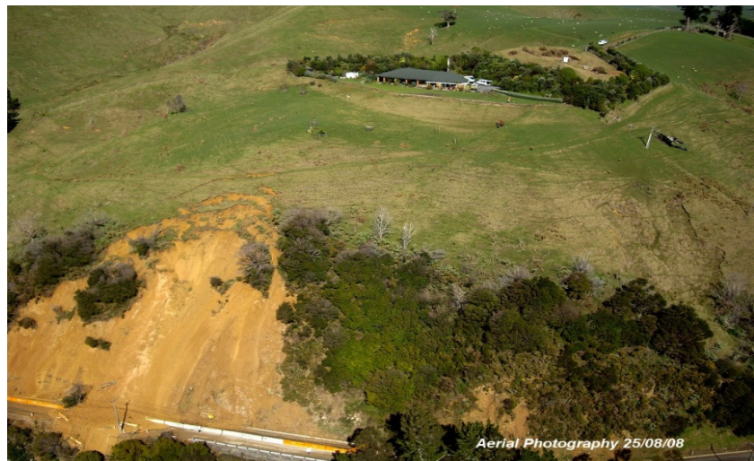
Figure 1: Road Slip Face August 2008
