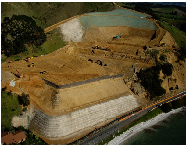
Figure 13: Toe Buttress Completion May 2009
