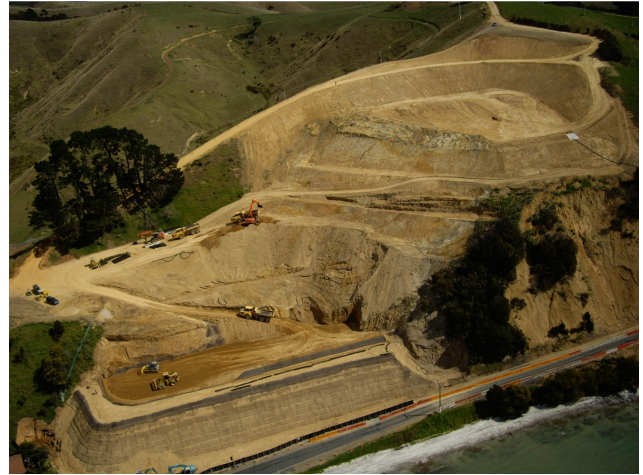
Figure 12: Toe Buttress Under Construction April 2009
