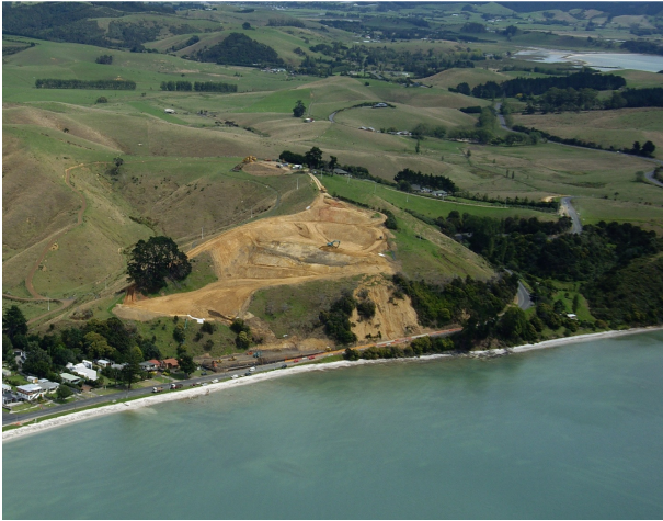
Figure 11: Earthworks and Bored Drainage March 2009
