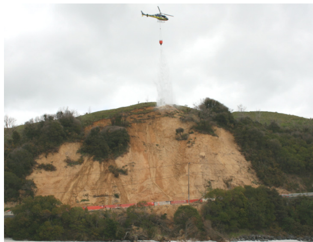
Figure 8: Sluicing in Progress
