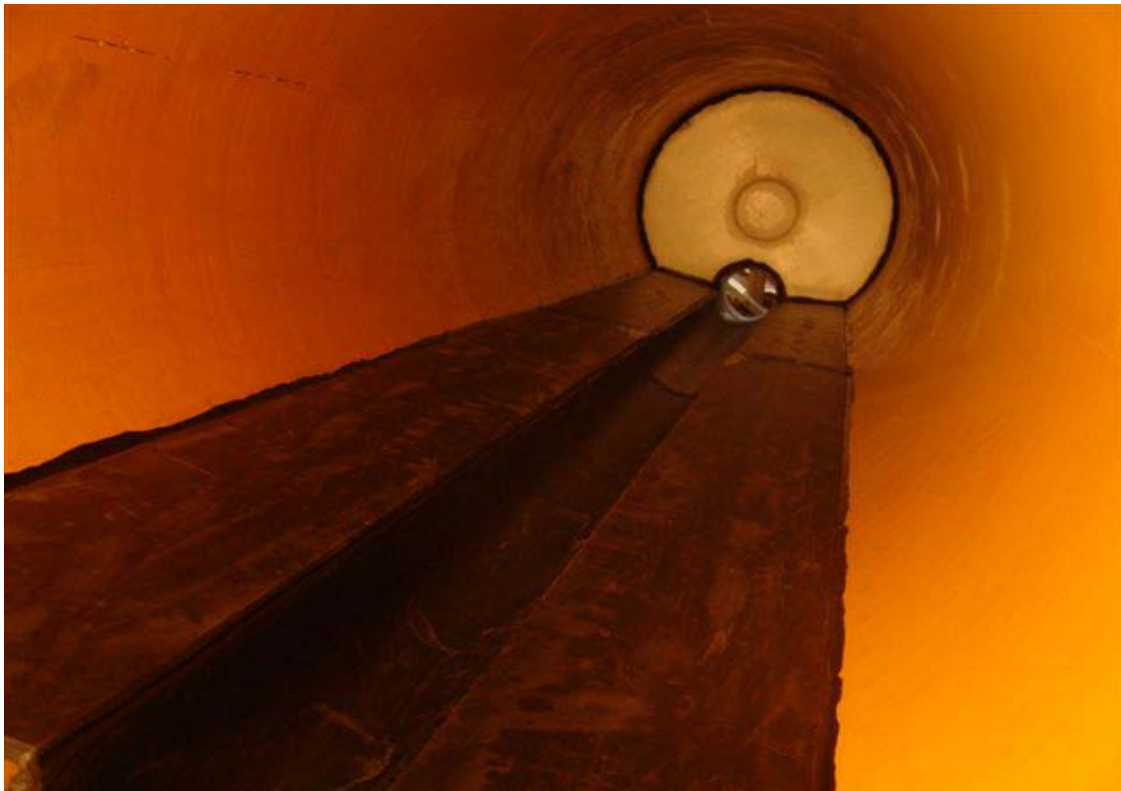
Figure 1 – Retention Tank, with 300mm Dia Dwf channel
