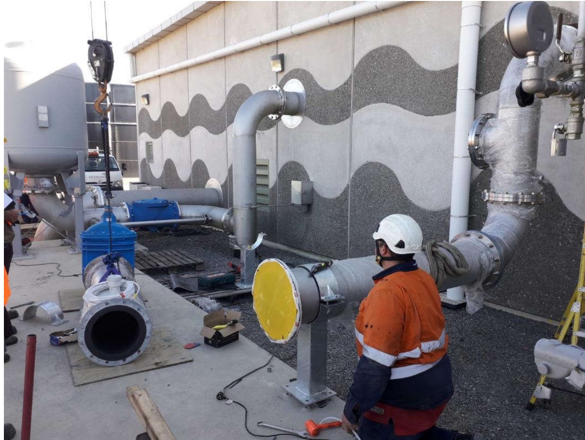
New headworks for Richmond West and South Trunk Main
