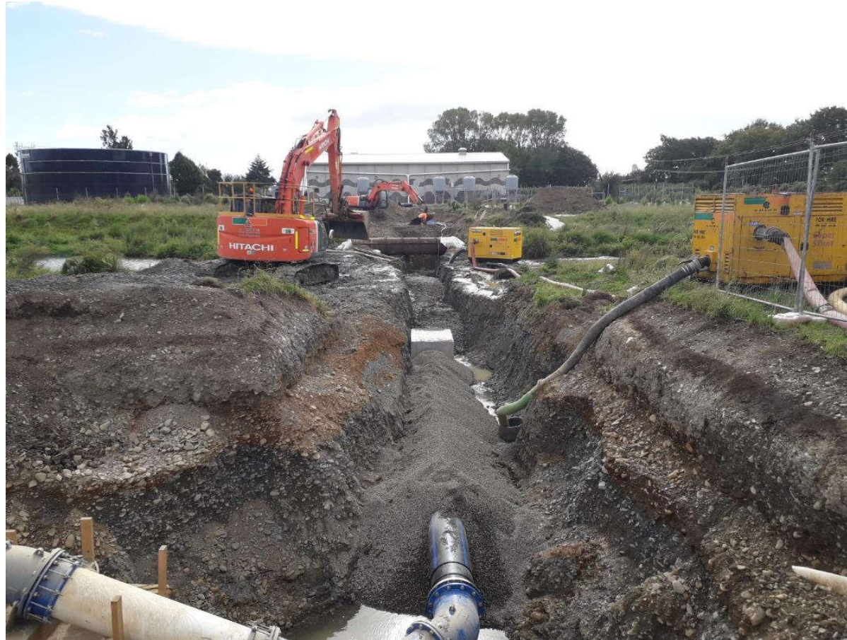
375mm dia trunk main crossing under Borck Creek
